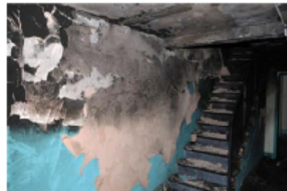
Stairwell opposite the scooter. Note: spalled plaster from the stairwell has fallen onto the stairs
