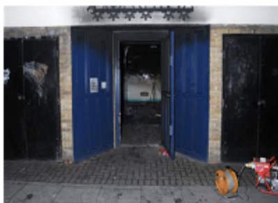
View of front communal entrance
