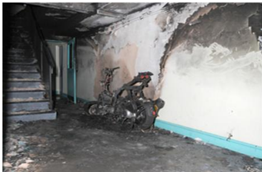
Clear burn pattern behind the scooter Note: rear tyre is still intact
